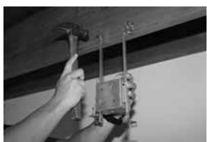
Step 1: Use the provided nails or wood screws to install to a wood joist
