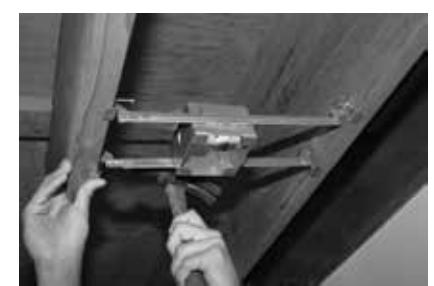
Step 3: Nail or screw to wood joist and adjust unit vertically or horizontally to ensure flush alignment
